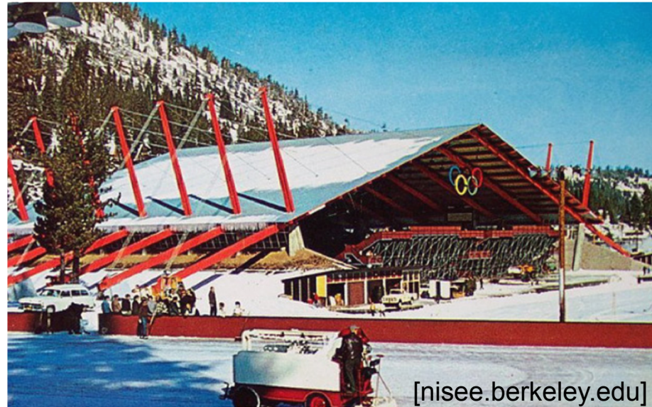
Blyth Arena- 1959 Squaw Valley, California 16-Mast Cable Stay 300 feet by 232 feet
